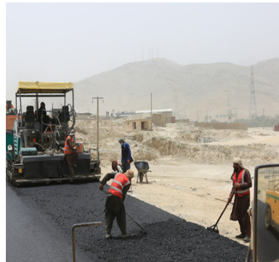
Road works in Kabul
