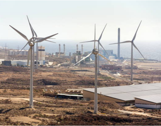
Wind turbine installation site
